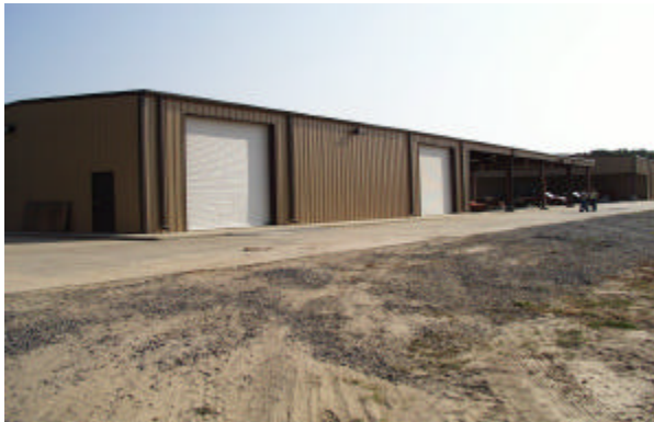
This is an example of a typical metal building erected by LAFA for the department. (Photo taken 8/29/00)
