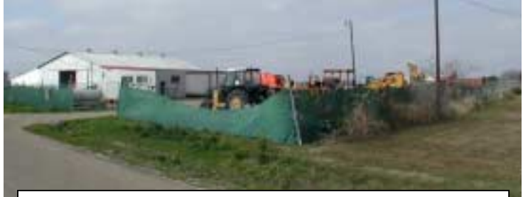
Opelousas maintenance yard that is located approximately 5 miles from three other maintenance yards
