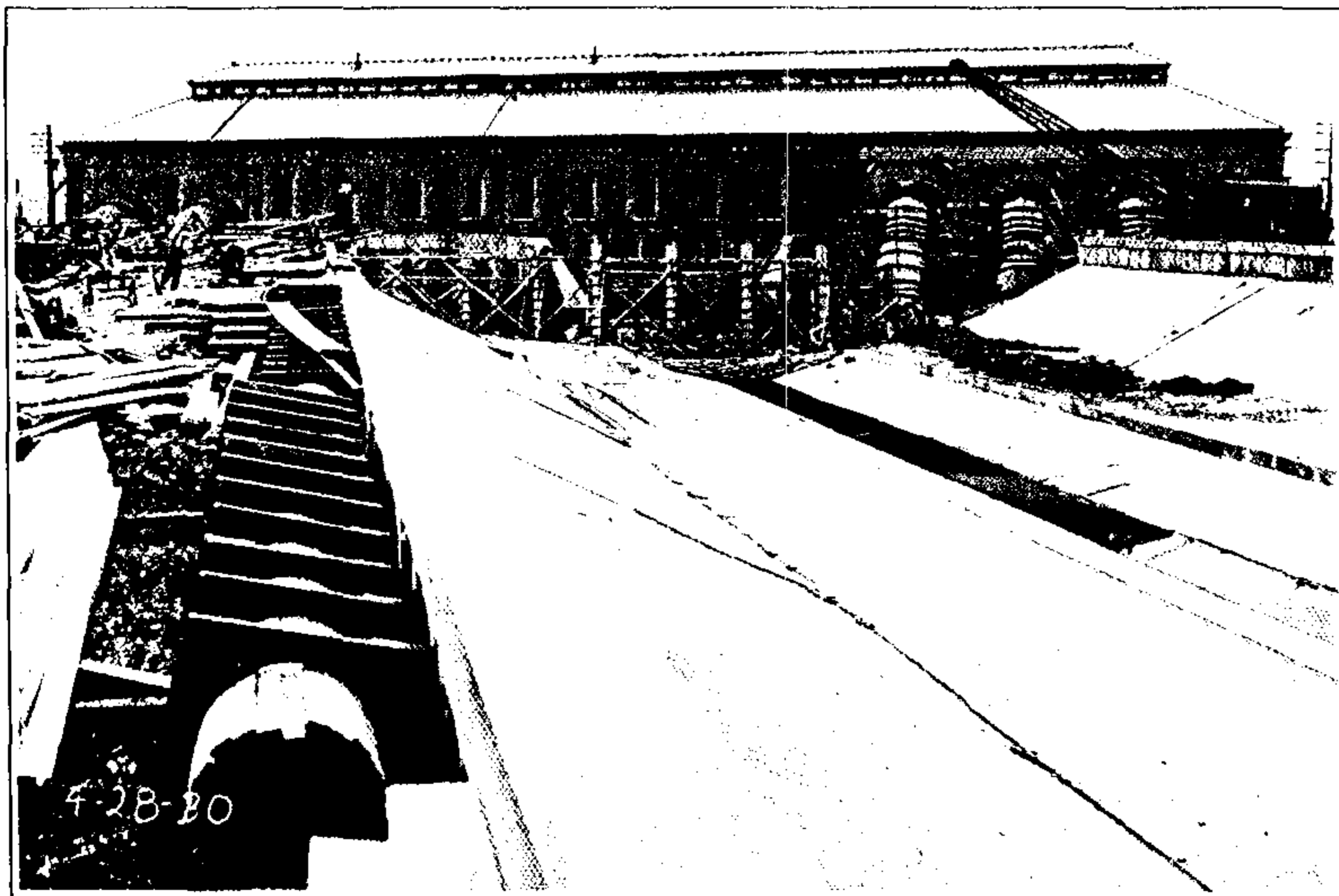
This 1930 photo of Drainage Pumping Station No. 1 shows work to enlarge the station and construction of the 16,000-foot-long Washington-Palmetto Canal, considered the "largest in the world."
