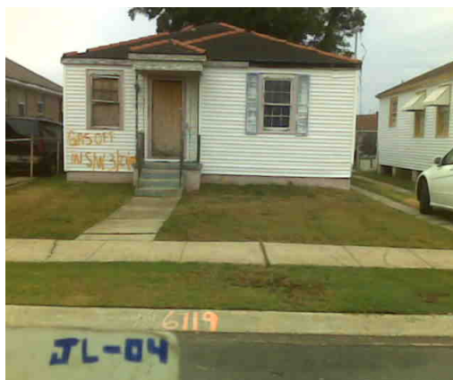
Before LLT Demolition
