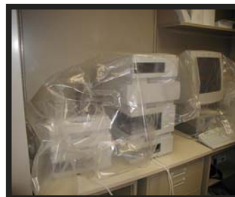
Equipment in Lab Affected by Moisture Problems in A. O. Williams Hall
